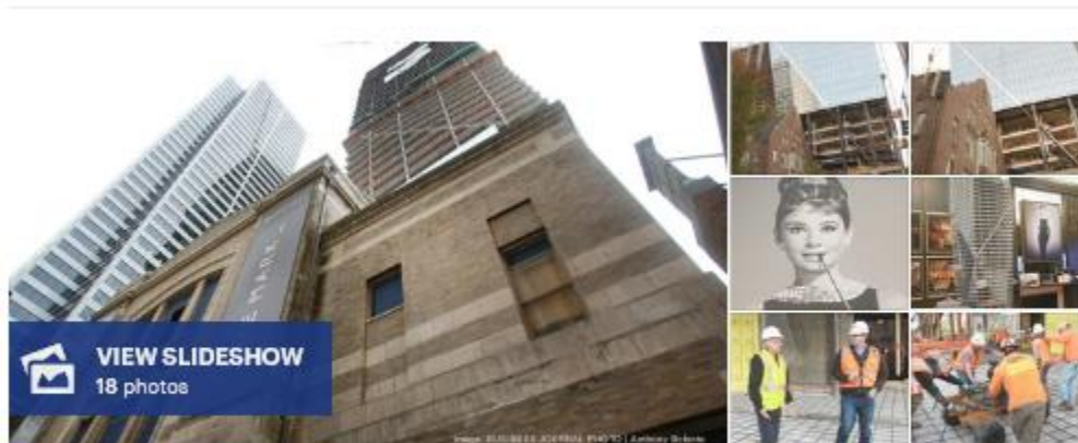
The Mark high-rise towers over the former First United Methodist Church, which is the... more
